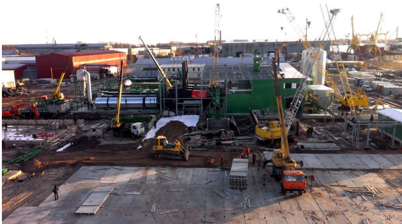
Arkhangelsk pellet mill construction site, November 21, 2013
