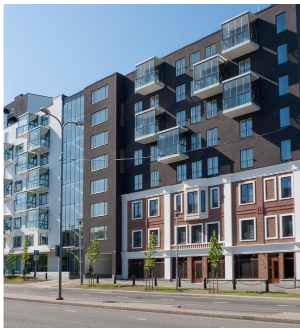
APARTMENT BUILDING AT TARTU MNT. 50A, TALLINN
