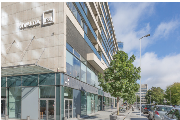
Vilnius Gates Business Centre Premises on Gyneju Street
