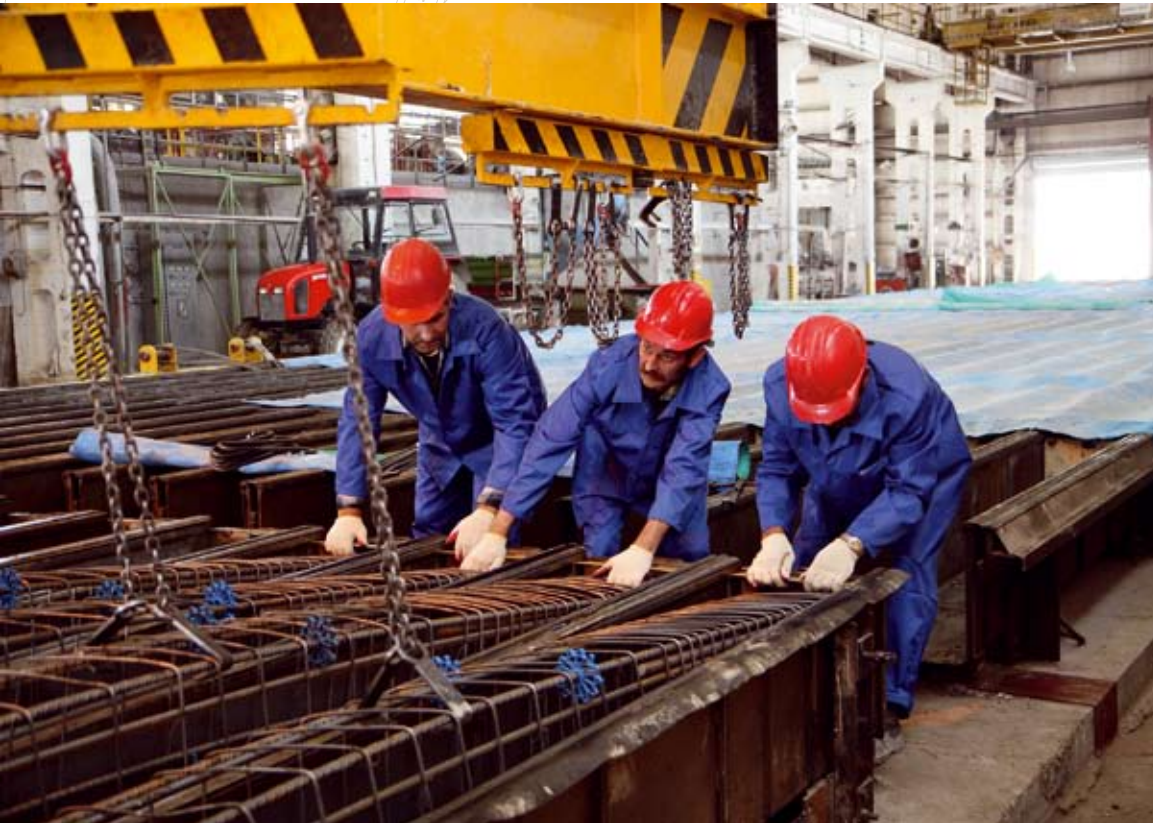
Aarsleff has invested in a pile factory in Poland. The factory now produces 150,000 rm of piles per year.
