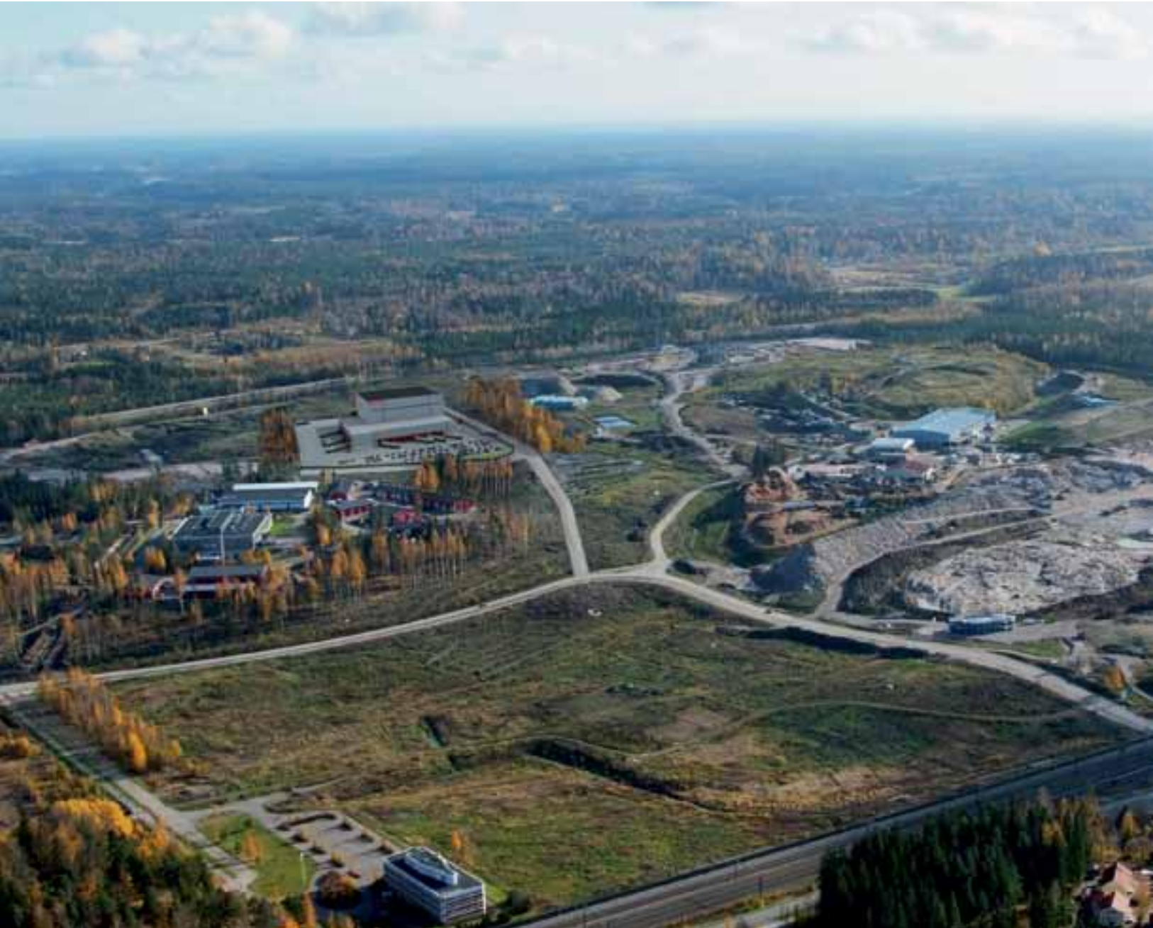
The construction of the Kerca logistics area will begin with Anttila's central warehouse. Kerca is a joint project of SRV and the City of Kerava.
