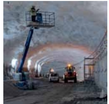
Helsinki City service tunnel, Helsinki
