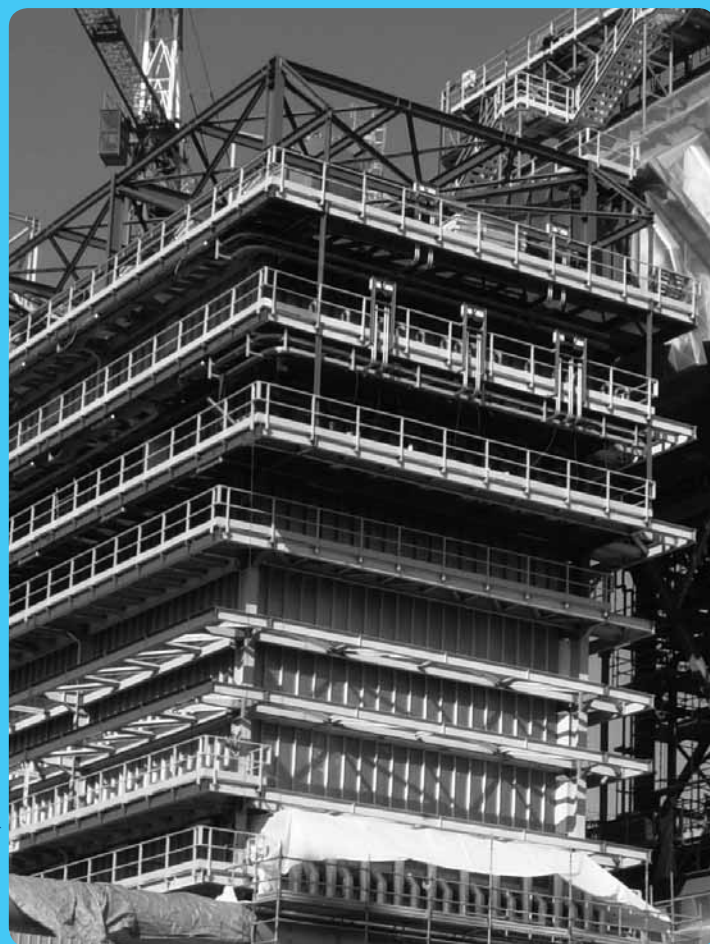
The first of Torrealvaldiga Nord's three absorber towers under construction.
