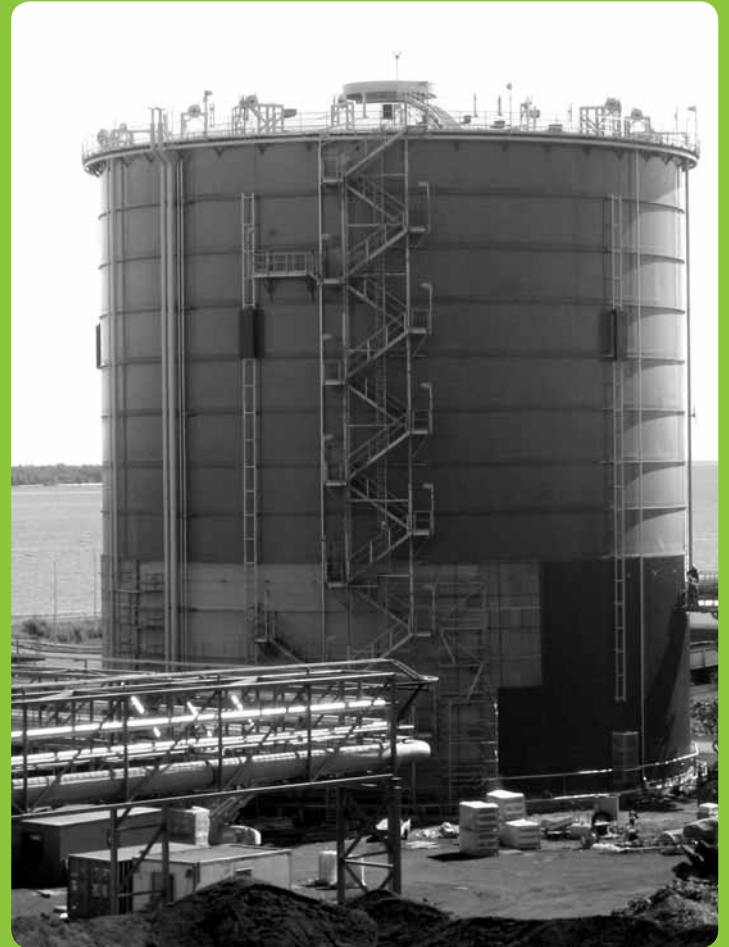
The carbon monoxide gasholder in Tornio.
