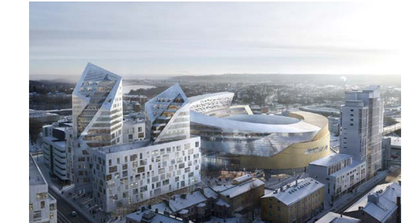
The Central Deck and Arena project will create a completely new part of the city on top of the railway tracks in the heart of Tampere.
