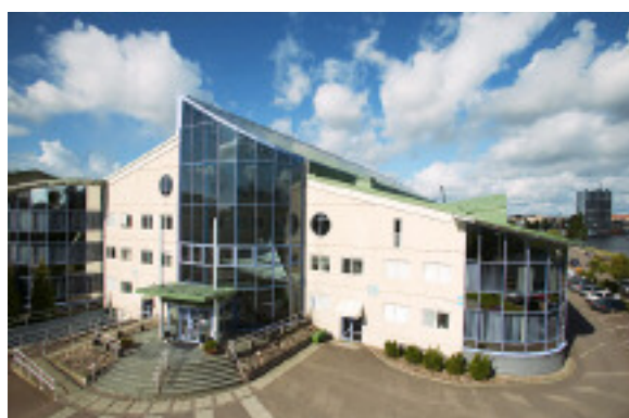
Barkassen 7. Vectura Consulting will move into the property Barkassen 7 in Karlstad during the first quarter of 2010.
