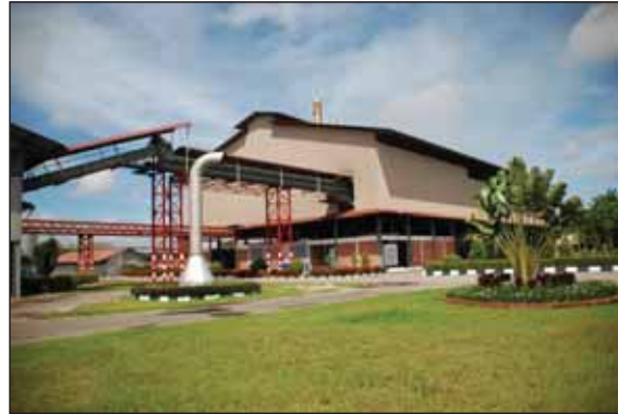
UP's "State of the Art" Biomass Reciprocating Boiler (BRB) at the Jendarata Palm Oil Mill Complex. The project is certified as a Clean Development Mechanism Project in accordance with the Kyoto Protocol with the objective to reduce Greenhouse Gas Emissions.
