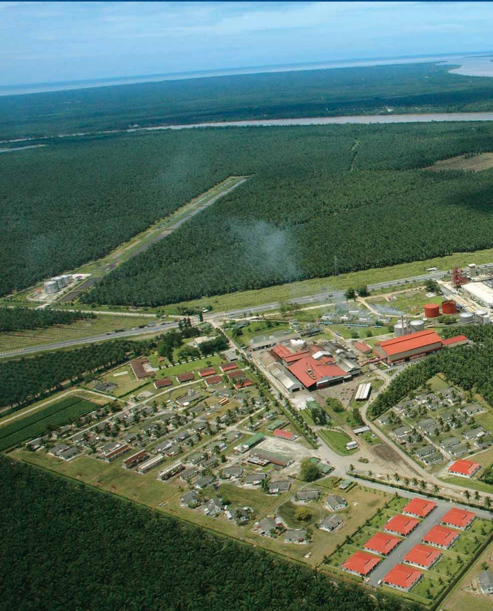
A helicopter view of Division 3, Jendarata Estate, showing its housing areas with its Palm Oil Mill and Unitata's Refinery Complex. The Bernam River is seen in the background.
