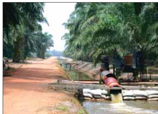
Water management activities within the estate.
