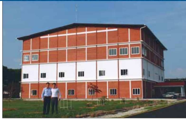
The newly constructed PKS Plant at Unitata Berhad. In the foreground are Ybhg. Dato' Carl Bek-Nielsen and Mr. Martin Bek-Nielsen.
