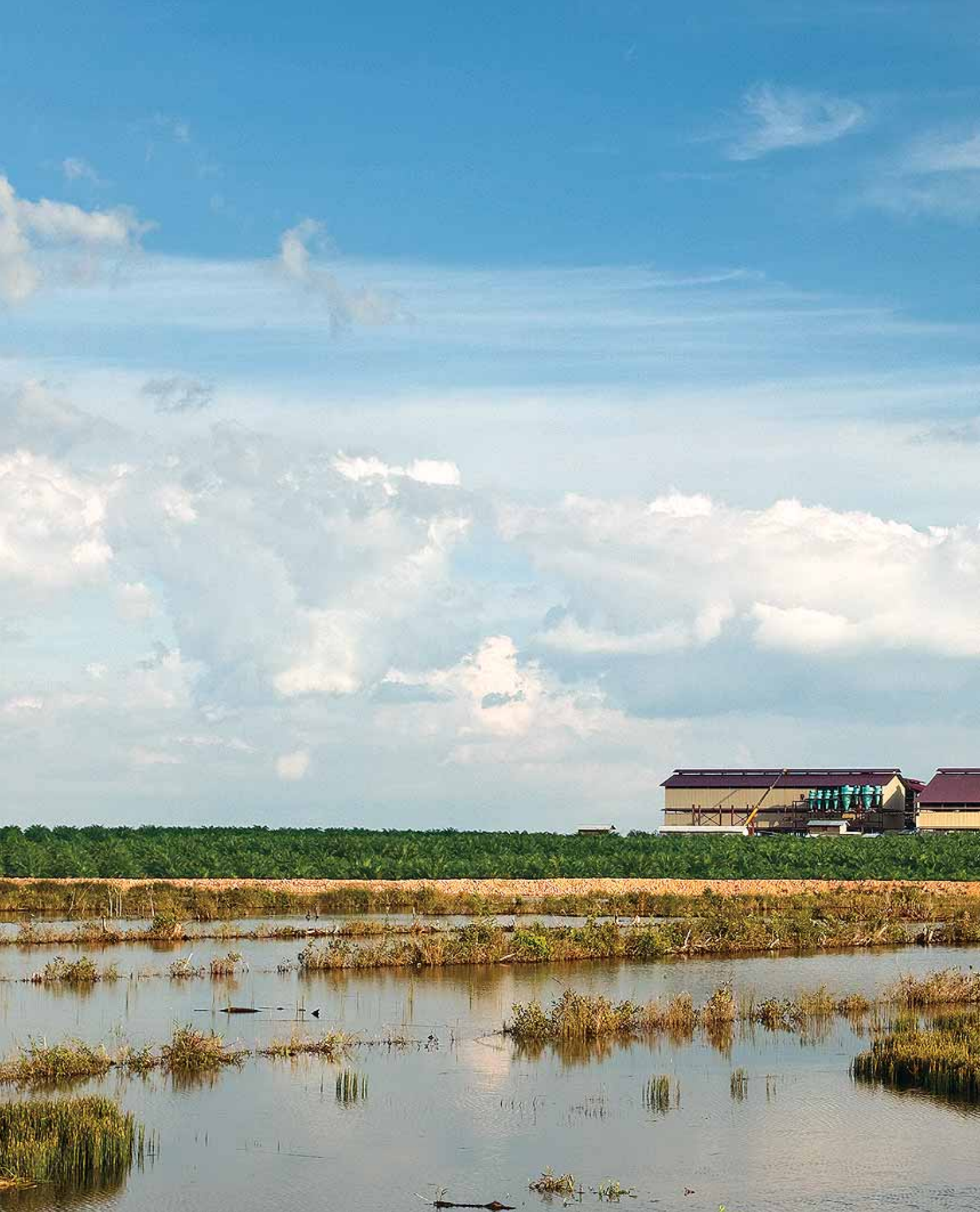
A reservoir with a water storage capacity of nearly 2 million cubic metres built to ensure uninterrupted water supply to the company's state of the art Palm Oil Mill at Lada Estate, Indonesia, in the background.
