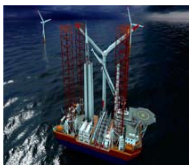
■ The Service Jack 2 installation vessel for the Sheringham Shoal Offshore Wind Farm
