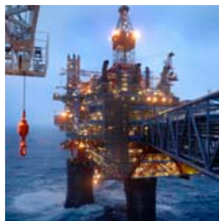
Sleipner A is an important hub for gas deliveries to Europe.
