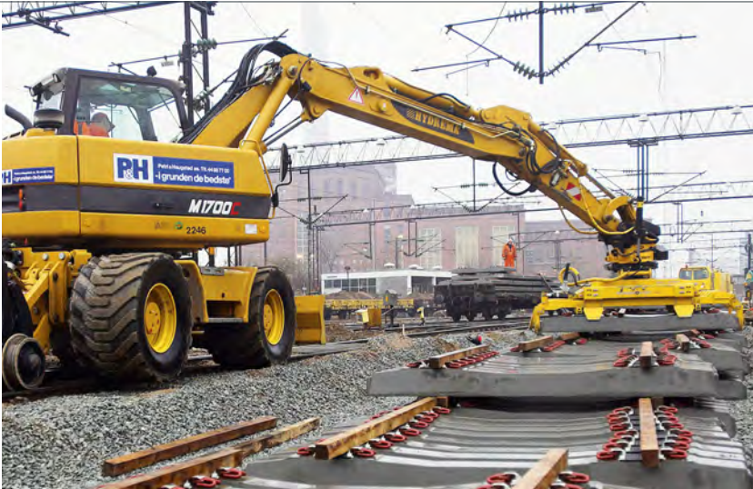
Renewal of depot tracks, Copenhagen.
