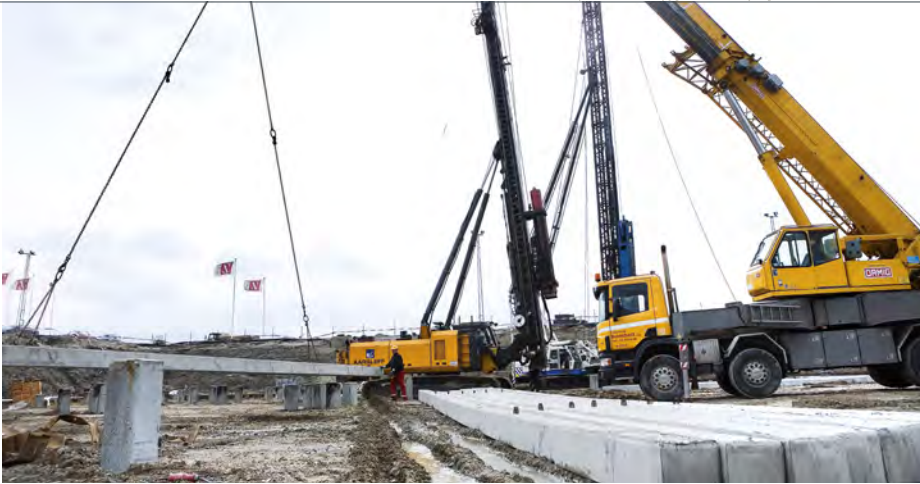
Piling, Z-House, Port of Aarhus.
