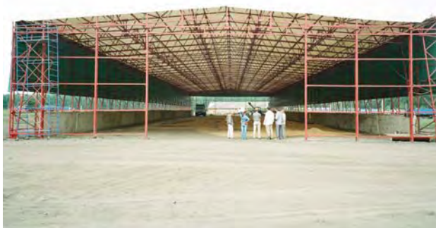
Hangar storage under construction in Tambov
