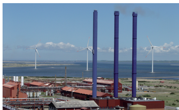
The combined heat and power plant at the factory in Denmark which is fuelled with natural gas.
