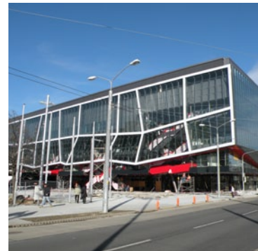
ONDREJ NEPELA ARENA, BRATISLAVA Systemair a.s, Slovakia, has supplied Frico air curtains for all entrances, duct fans and air distribution products for all ventilation for the main arena for the 2011 Ice Hockey World Championships. The arena first opened back in 1940 and was renovated in 2011. At the same time, its capacity was raised to 10,000 spectators.
