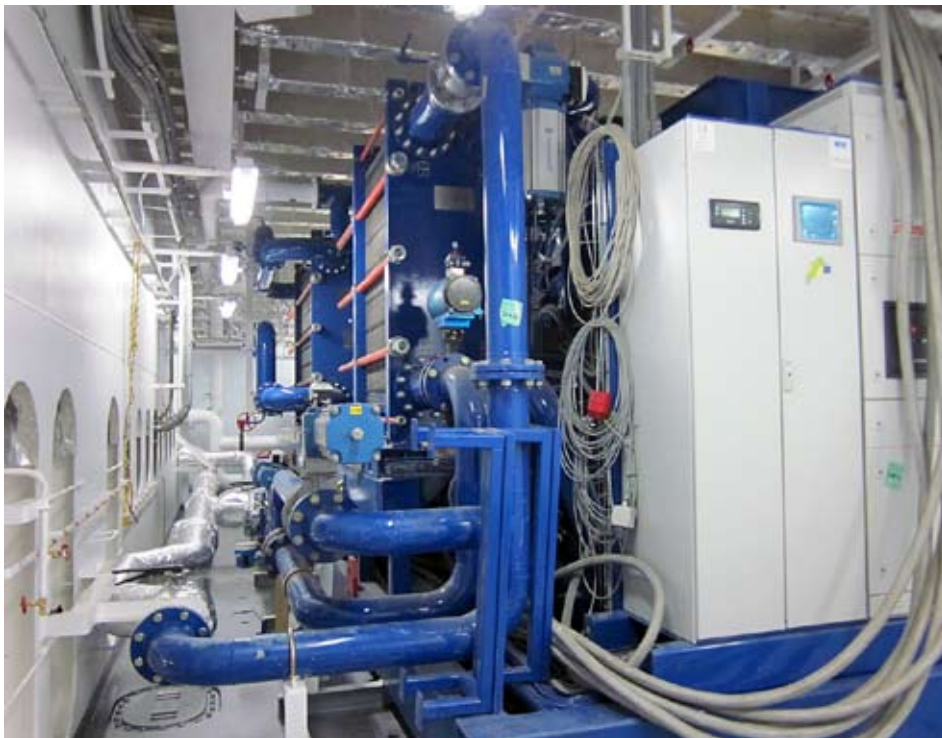
An Opcon Powerbox unit being installed onboard a Wallenius LCTC vessel.
