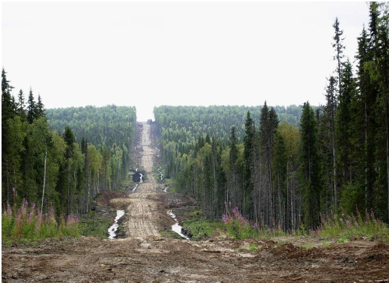
Road construction in the Arkhangelsk Region
