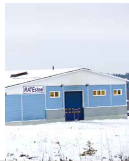
The RATEsteel Oy facilities will be expanded in 2008.
