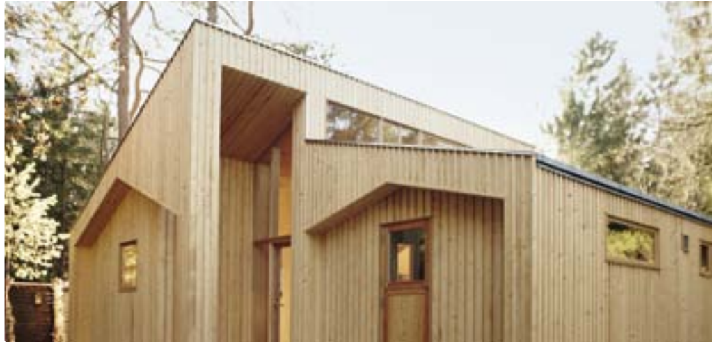
A house made by Danish architects from UPM's spruce plywood provides a new model for sustainable building.
