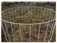
Exel Composites supplied six identical experimental 'arrays' inside the forest. Each array is served by a permanent tower crane and comprises 32 CO<sup>2</sup> vent masts 28 metres high in a 25 metre circle, surrounding a group of old-growth trees. The vent structure is fabricated from pultruded glass-fibre composite material.
