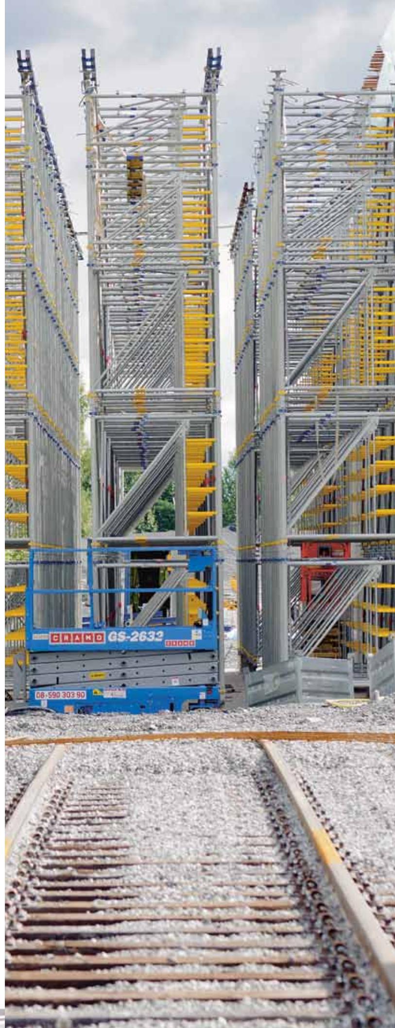
Construction of the railway terminal with loading hoppers continued throughout 2011.
