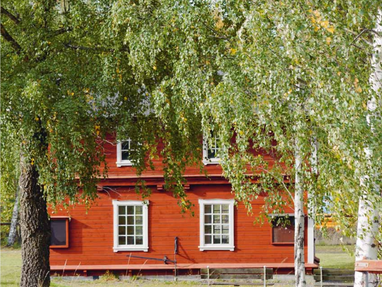
The old pump house at Storrymningen.
