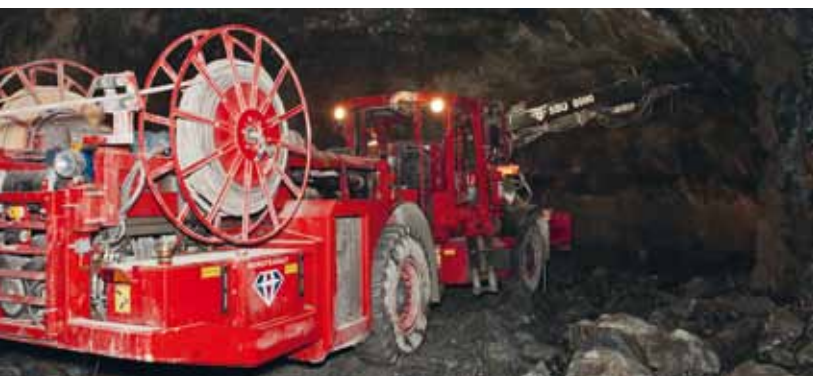
Mechanical scaling after blasting
