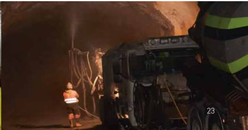
Shotcreting of the drift roof to increase safety.
