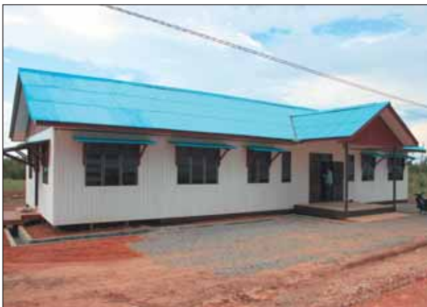
The completed temporary office building fully furnished and ready to be occupied.
