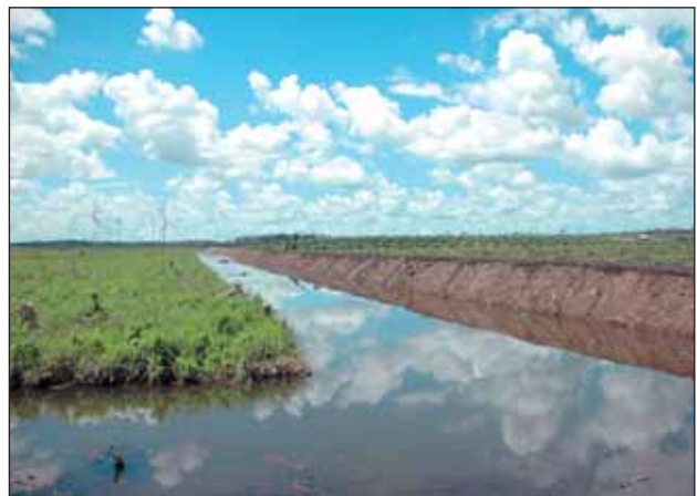
The reservoir with its large bund is situated beside the mill site. The total water retention capacity is 1.5 million m 3 .
