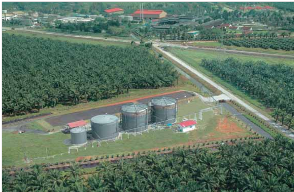
An aerial view of the Biogas Digester at Jendarata Estate which is certified as a Clean Development Mechanism Project enabling the mill to generate biorenewable energy from the Palm Oil Mill effluent.
