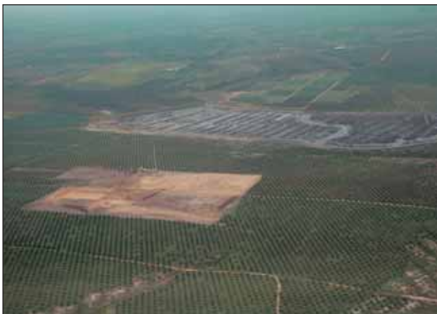
In the foreground the mill site is being prepared, with a large water reservoir in the background which will ensure sufficient water supply to the future Palm Oil Mill at Lada.
