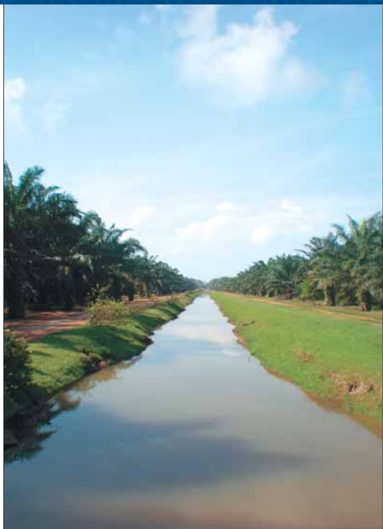
Water management and good drainage systems are critical in oil palm cultivation to maximize yields.
