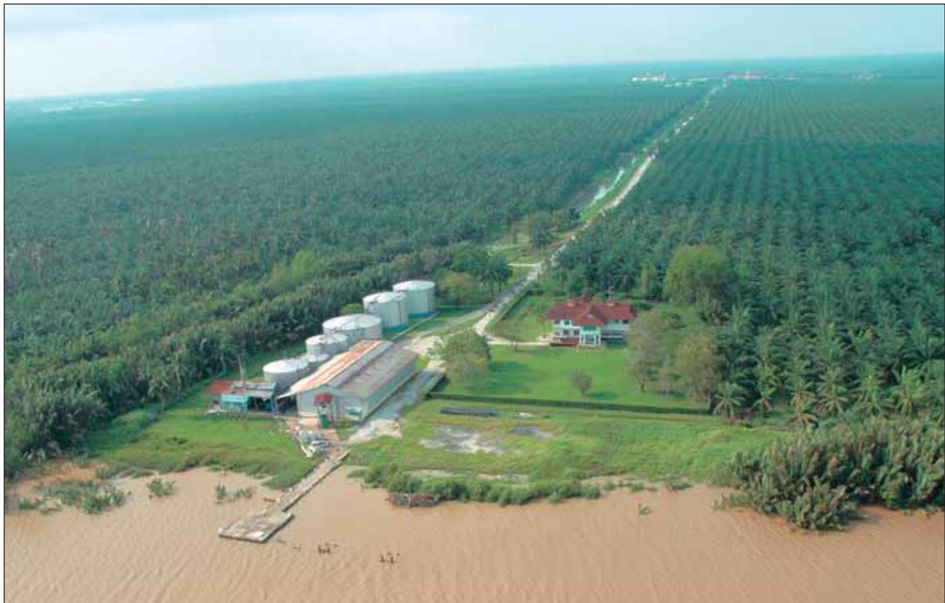
Bulking installation at Jendarata Riverside with the Bernam River at the foreground.
