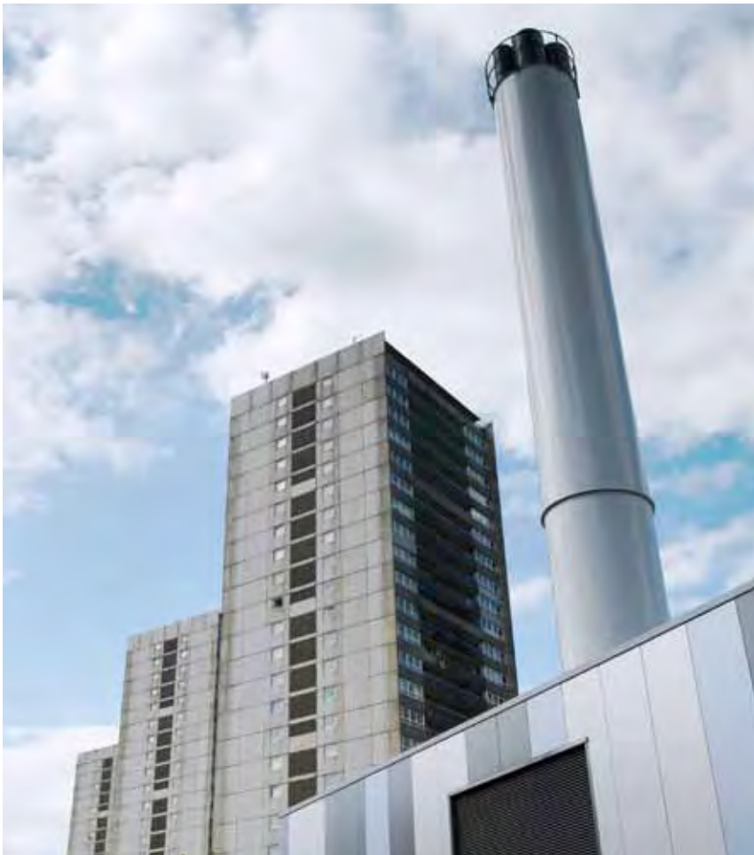
The Danish subsidiary KVM has supplied district-heating equipment for a large-scale project in Scotland to replace conventional electric radiators in the more than 1,500 homes on the Wyndford Estate built in the 1960s. Now residents can look forward to lower heating costs and a reduced environmental impact, thanks to a dramatic fall in the properties' carbon dioxide emissions.
