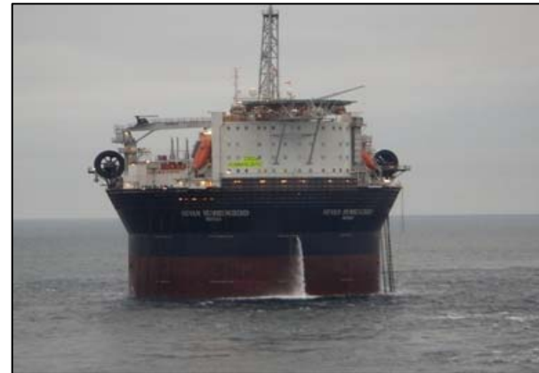
December 2007 – Hummingbird installed
