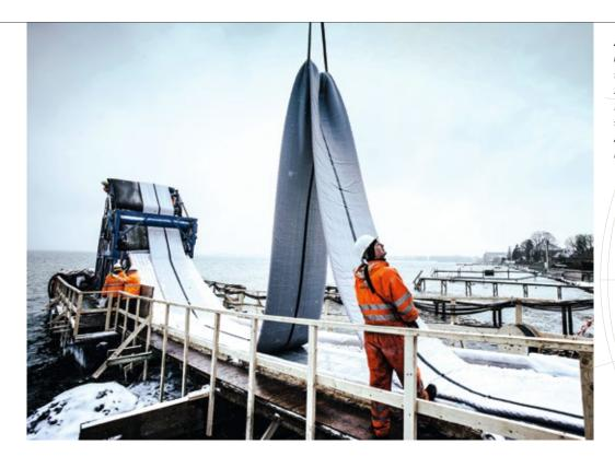
Aarsleff renews outfall in Oresund. A total of 1,100 metres in the dimension DN1250 mm, The installations took place from a temporary bridge which was able to withstand a pressure of up to 20 tons.
