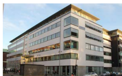
Gullbergsvass 5:26, "Tennet", Kilskatan 4, Gothenburg.
