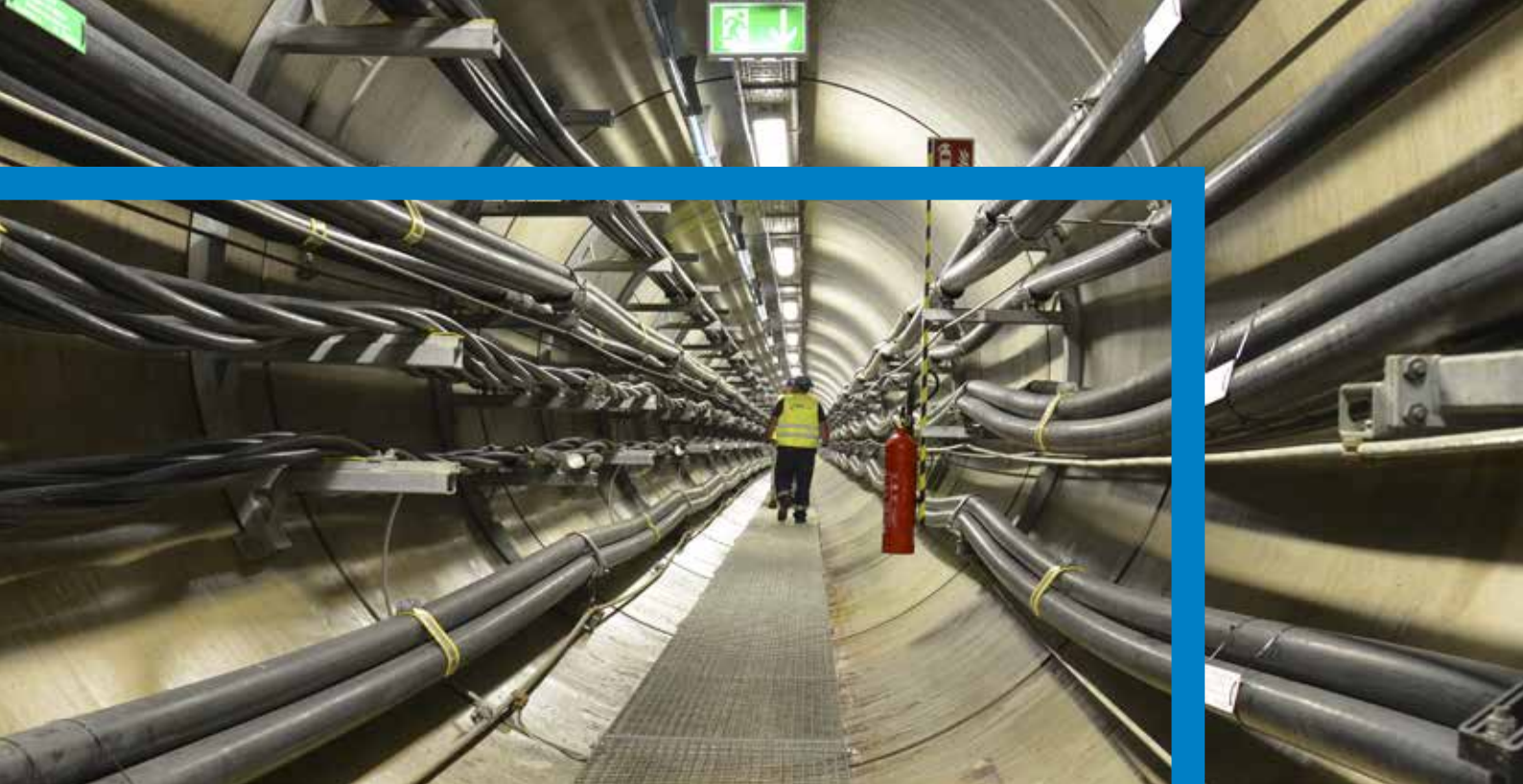
Luxembourg tunnel project incorporating a wide selection of power cables
