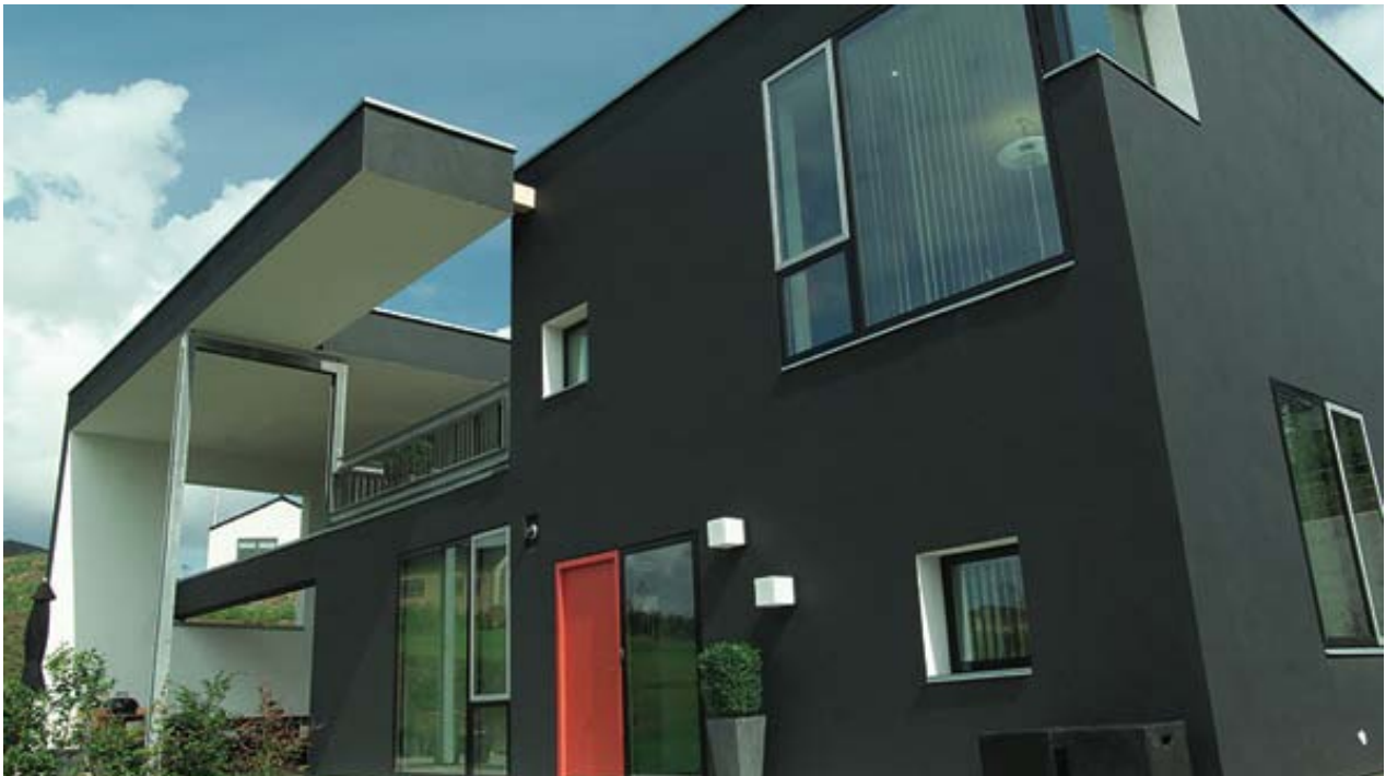
Exclusive home built of solid blocks from H+H.
