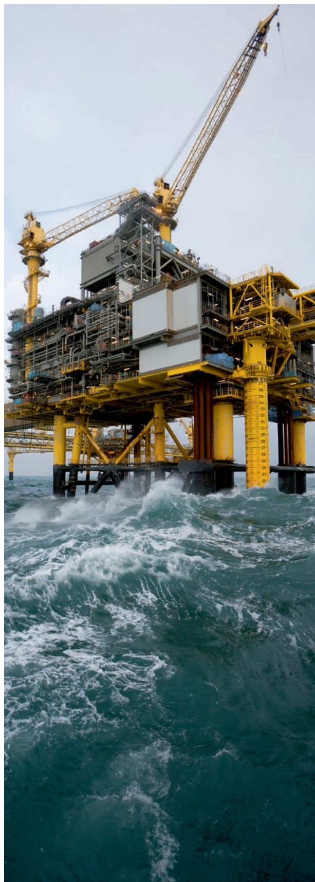
Maersk Oil's platforms in the North Sea are built to endure extreme weather conditions.
