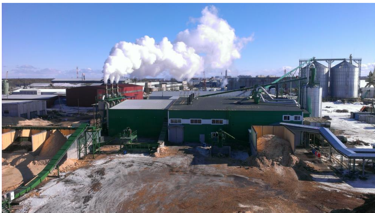
The Company's newly constructed pellet mill in Arkhangelsk, March 2014 (with all three presses operating as can be seen from the chimneys)
