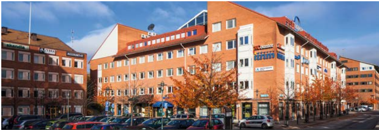
SVÅRDET 7, DANDERYD Office and retail property in the prime billboard location next to the E18 with good communication links and a large range of services. The property, which was taken over in December 2013, adjoins Mörby Centrum metro station. Kungsleden owns a further three office properties in Danderyd. Total lettable area is 100,000 sq. m.
