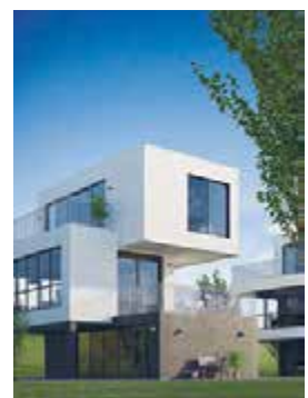
Lindab's solutions in tomorrow's buildings.
