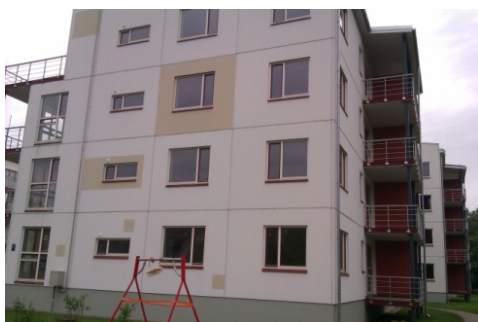
Bisumuiza's penultimate apartment building as at 30 May 2013.
