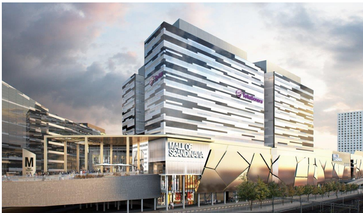
In April, Fabege and TeliaSonera signed a contract for the leasing of the entire Scandinavian Office Building in Arenastaden, Solna. TeliaSonera will relocate to the property in spring 2016.
