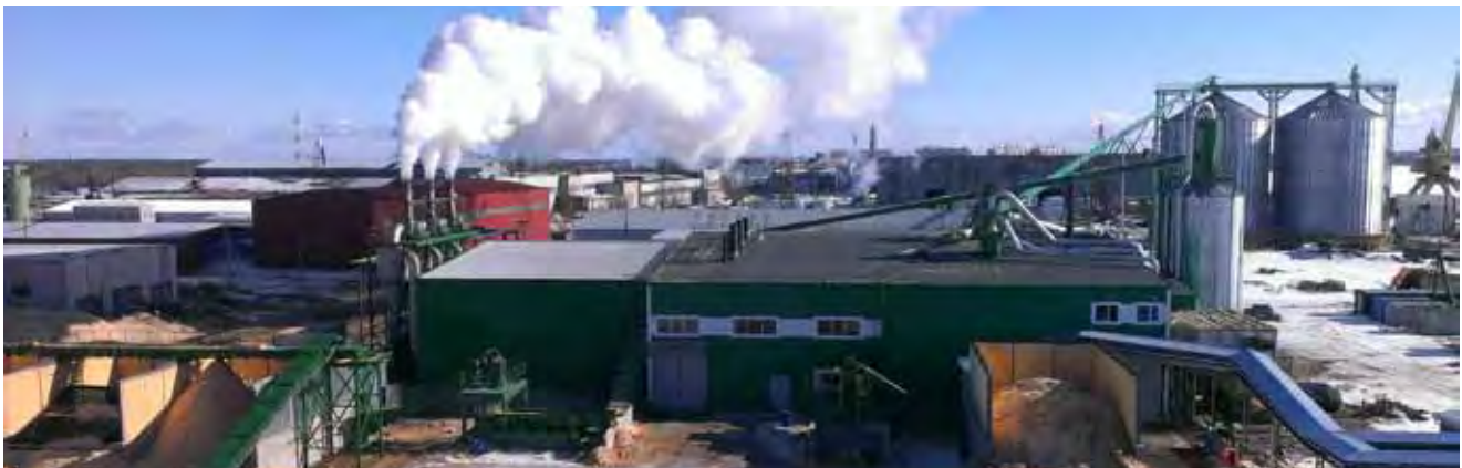
The Company's new pellet mill in Arkhangelsk
