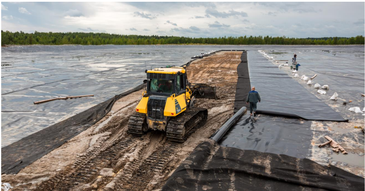
THE CLOSING OF INDUSTRIAL WASTE AND SEMI-COKE LANDFILL IN KOHTLA-JÄRVE CONTINUES IN 2014
