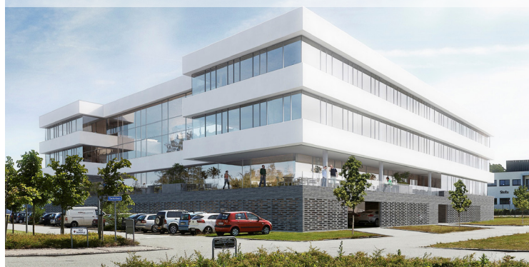
Alfa Laval, office building, Aalborg, Denmark
