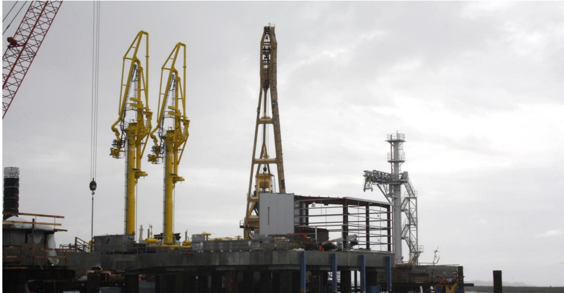
Jetty service platforms construction
