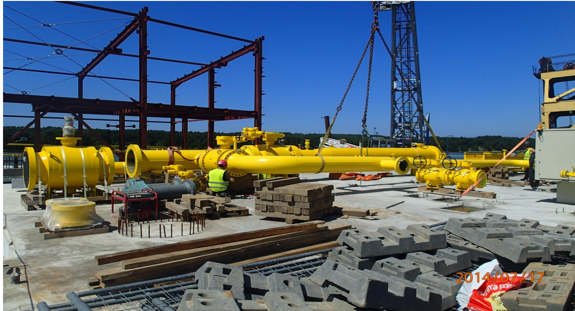
Finished gas metering station construction
