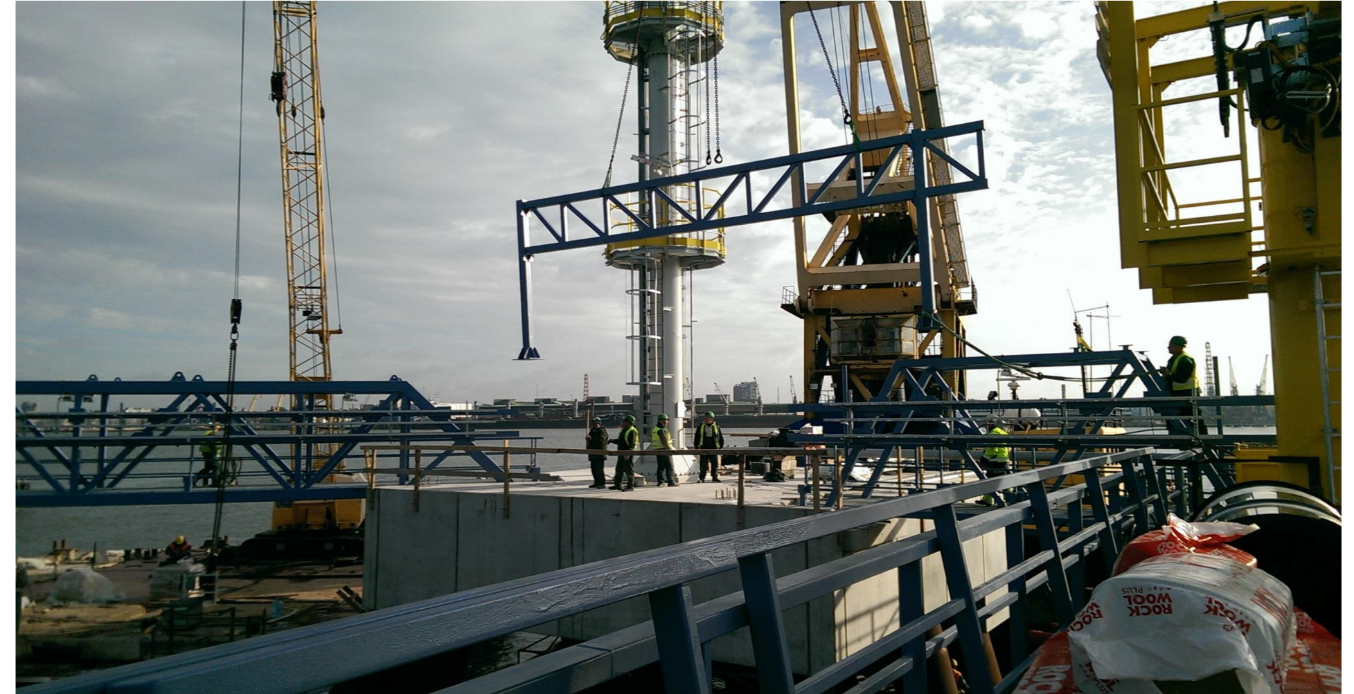
Jetty supports construction
