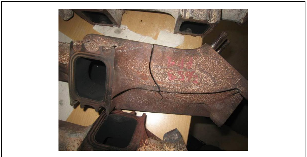
figure 10-13: Crack in the manifold between the turbocharger and the rear cylinder (PROSE)
