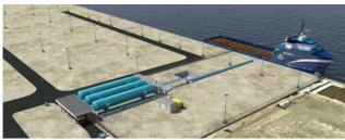
**9.7.** Wärtsilä contracted to supply control system for Harvey Gulf's shore-based LNG fuelling facility - the first source of LNG fuel in the Gulf of Mexico.
