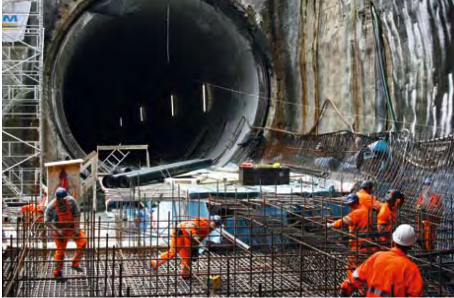
Station Triangeln, Citytunnel Malmö.
