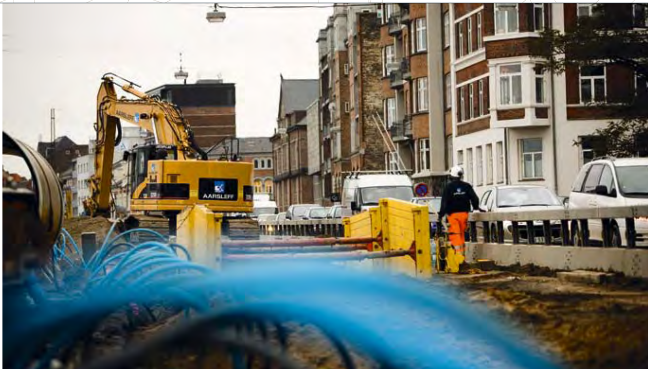
Sewer rehabilitation, Kystvejen, Aarhus.
