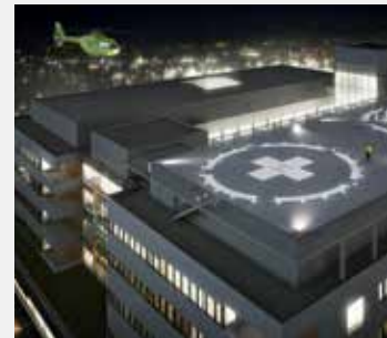
The most serious cases can be taken care of via the rooftop helipad.
