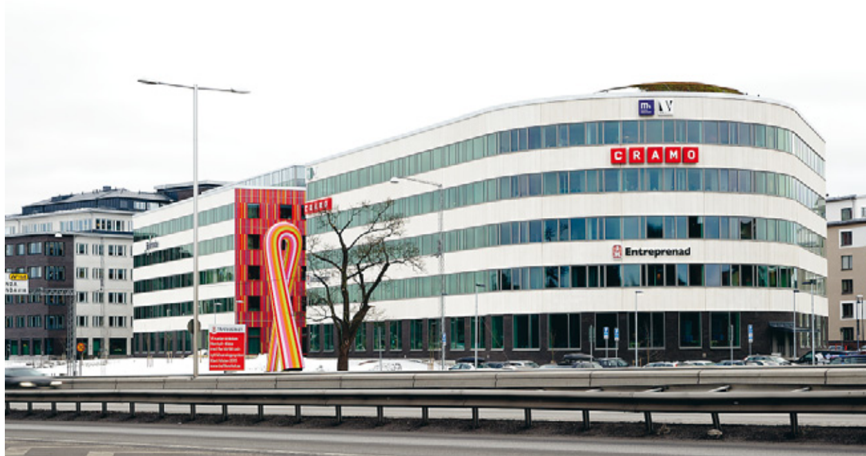
JM Entreprenad's new office in Frösunda Port, Solna.
