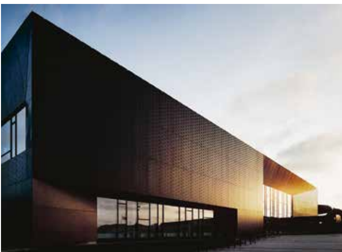
Public baths that play with light. The aspiration for the Swedish city of Ystad's new public baths was a building that would stand out aesthetically as well as functionally, without overburdening the municipal budget. Sweco's architects worked with their partner in the project to bring a "Reflection"-themed building to life. The facade creates an intriguing interplay with light, with the building changing character throughout the day. Inside, visitors are greeted with family and competition pools in surroundings with large windows overlooking a nearby park.
