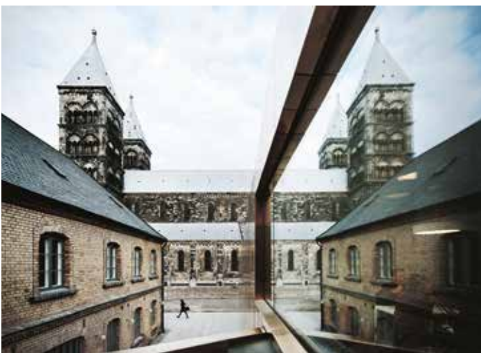
Ancient Swedish church smartens up with 3D. Buildings in smart cities produce information about themselves, facilitating maintenance and management. And this doesn't only apply to new buildings. Lund Cathedral, built in the 12 th century, is now equipped with the same technical potential. Sweco produced a 3D visualisation of the church that can be used for everything from changing pipes to forecasting the church's capacity to manage climate change.
