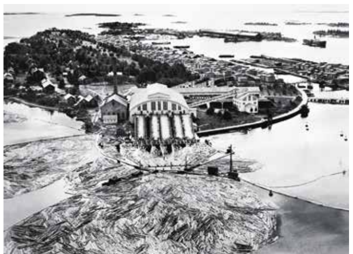
Contaminated historical environment freed from toxins. A sawmill on Norrbyskär in northern Sweden's municipality of Umeå spread toxic substances over large areas in the early 1900s. The island, of cultural-historical value, will now be decontaminated. Sweco has been commissioned to examine the ground and propose remedial measures to clear it of toxins.
