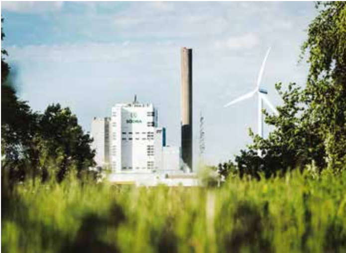
Record investment by forest industry. The expansion of southern Sweden's forest owner association, Södra's, Värö pulp mill is currently one of the industry's largest investments. Sweco has been commissioned for the entire construction design project and will work with experts in a variety of areas. The mill will be one of the world's largest for needle-sulphate pulp.
