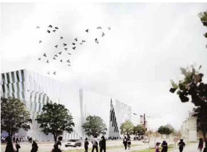
An office building for the future. When Finnish financial group OP Pohjola was planning a new office complex with space for 3,000 employees, they wanted to create a world-class working environment. Rather than building a traditional skyscraper, they preferred a campus-like area spread over 65,000 square metres. Sweco is behind the structural design of the innovative office building, which was awarded first prize at the 2014 Tekla Global BIM Awards.
