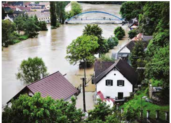
Czech Republic manages floods with map data. All EU countries are responsible for systematically mapping the risk of lake and river flooding. The Czech Republic has been hard hit by flooding in recent years. Sweco used GIS analysis to help the country plan measures to reduce the risk of future floods. Following completion of the project, there is now a comprehensive database of the greatest flood risk areas in the Czech Republic.
