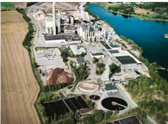
More paper pulp of higher quality. Pulp supplier Södra Cell is pursuing an initiative in Karlshamn, Sweden that will increase the capacity and quality of pulp production. Sweco is responsible for sub-project management and designing and planning the plant's reconstruction. To streamline this work, Sweco developed a 3D model that provides a comprehensive picture of the mill's needs and possible solutions.
