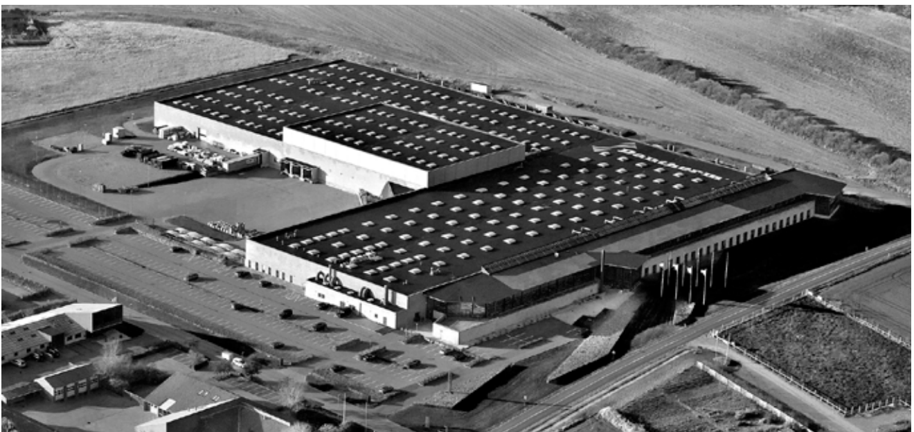
Dantherm's headquarters and production facilities in Skive, Denmark
