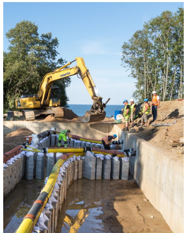
ESTLINK 2 CONSTRUCTION WORKS COMPLETED IN 2014.
