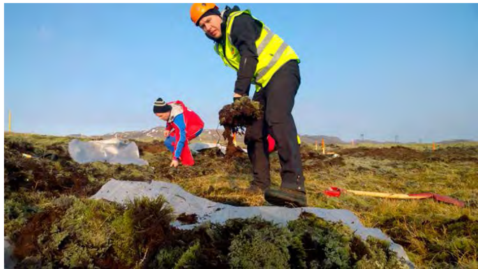
Search and rescue teams collect moss in the construction area of the Hverahlíð Pipeline
