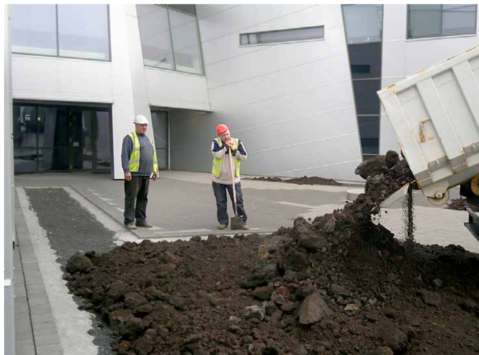
Figure 37. Moss and scoria from Hellisheidi utilised for the finishing of the entrance to Hellisheidi Geothermal Power Plant. Photos: Magna Magnúsdóttir.
