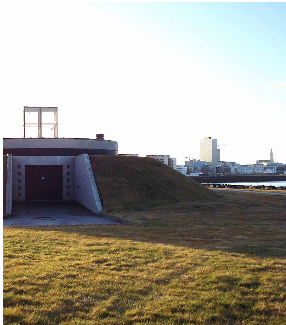
Figure 13. Pumping station at Laugalaekur. Photo: Thorsteinn Ari Thorgeirsson.
